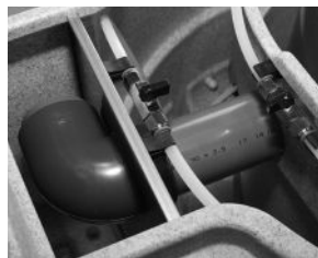
Figure 17.3 - By-pass in operation
