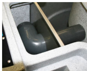
Figure 17.3 - By-pass in operation
